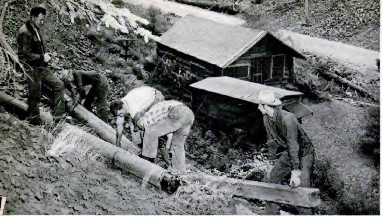
Beside an old cabin of a gold prospector, a new pipe line is laid for the Idaho mine now producing cobalt
